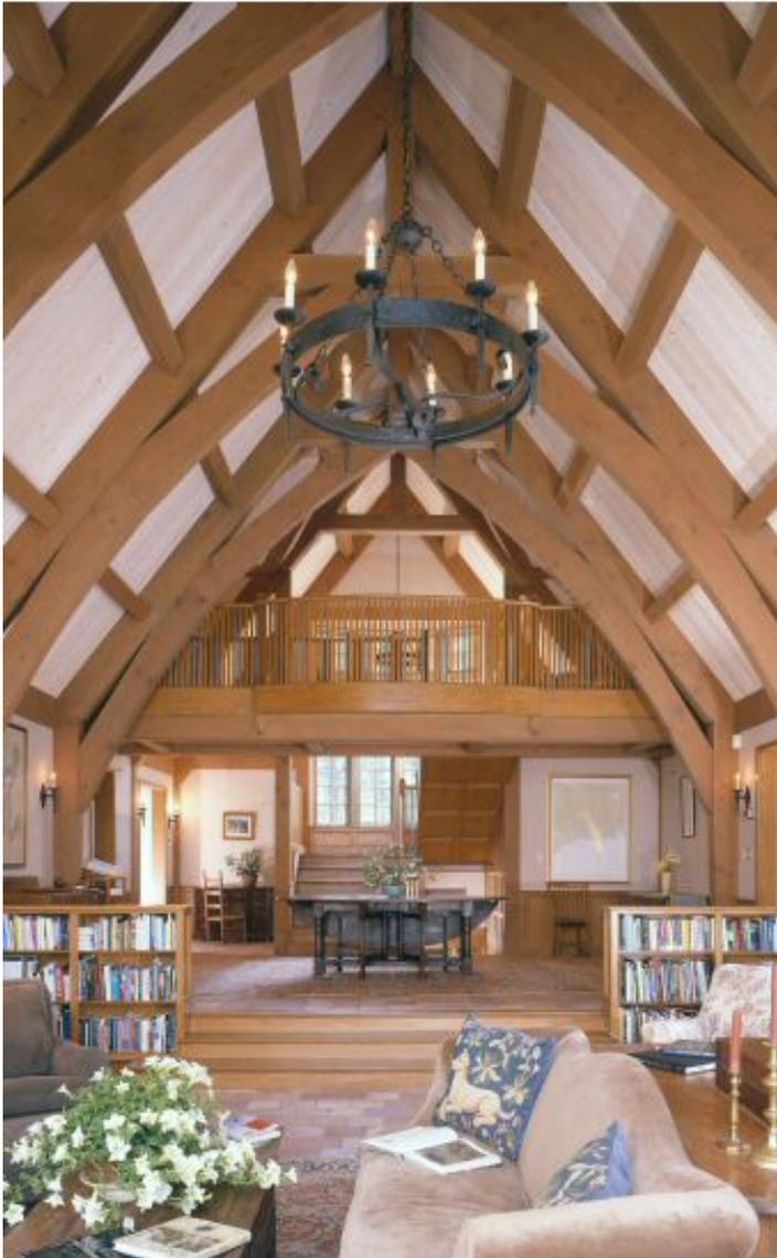
**Below: The frame, with its cruck-style trusses, was manufactured by Timberpeg East at their plant in Claremont, New Hampshire. The frame was constructed out of Douglas fir and then given a clear natural finish to fit in with the simple look of the frame.**
